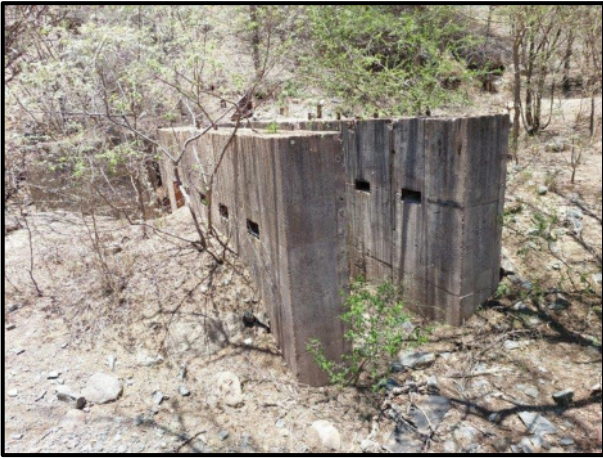
Figure 7.6. Foundation remains at RV003.
