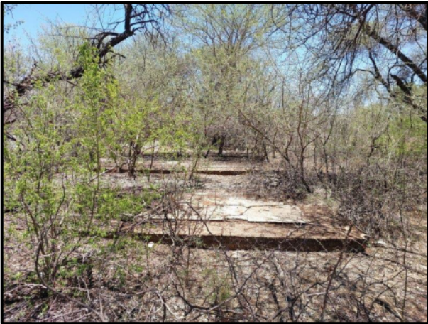
Figure 7.8. Foundation remains at RV004.
